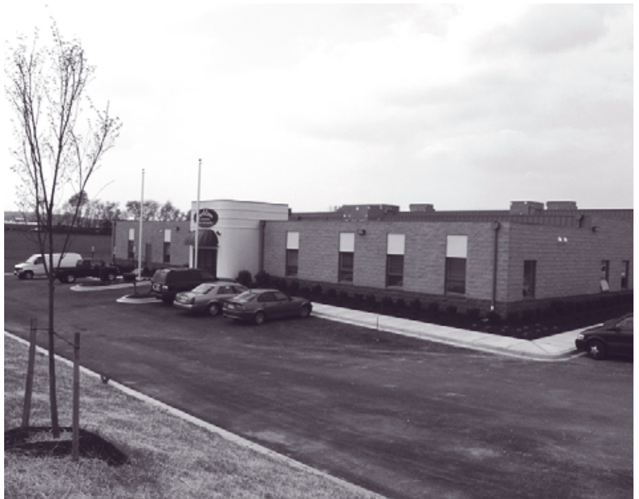
Integral Component's new 20,000-square-foot facility in the West Branch Trade Center in Westminster
